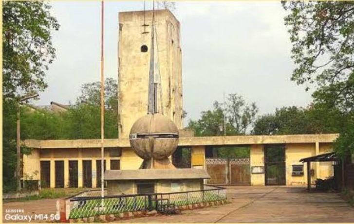
M.A.M.C. Factory (Main Gate)
